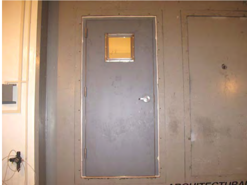
Receive Room View of the Installed Specimen
